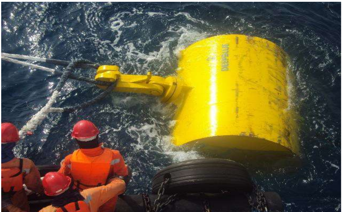
Figure 6 Installation of the Buoys and VERSATILE MOORING SYSTEM
