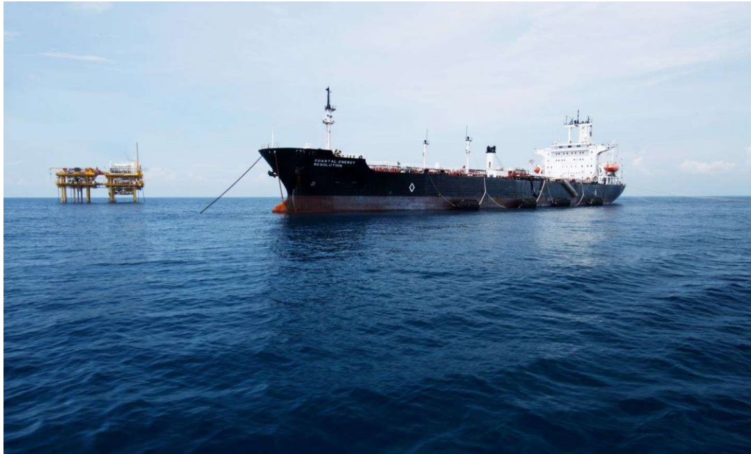
Figure 1 Tanker Moored with the VERSATILE MOORING SYSTEM and in production in the Gulf of Thailand
